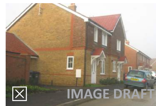
Secondary materials (tiles) poorly integrated on the facade
