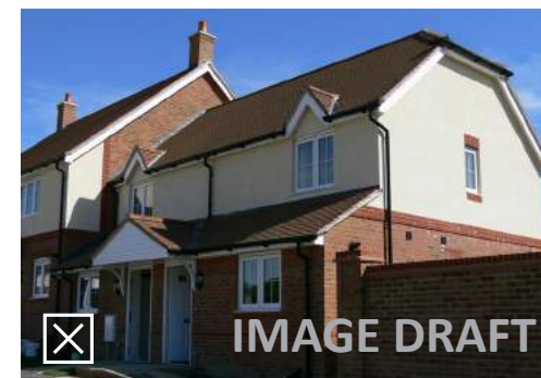
Poorly integrated porch and ground floor window projection which appear as 'bolt on' features
